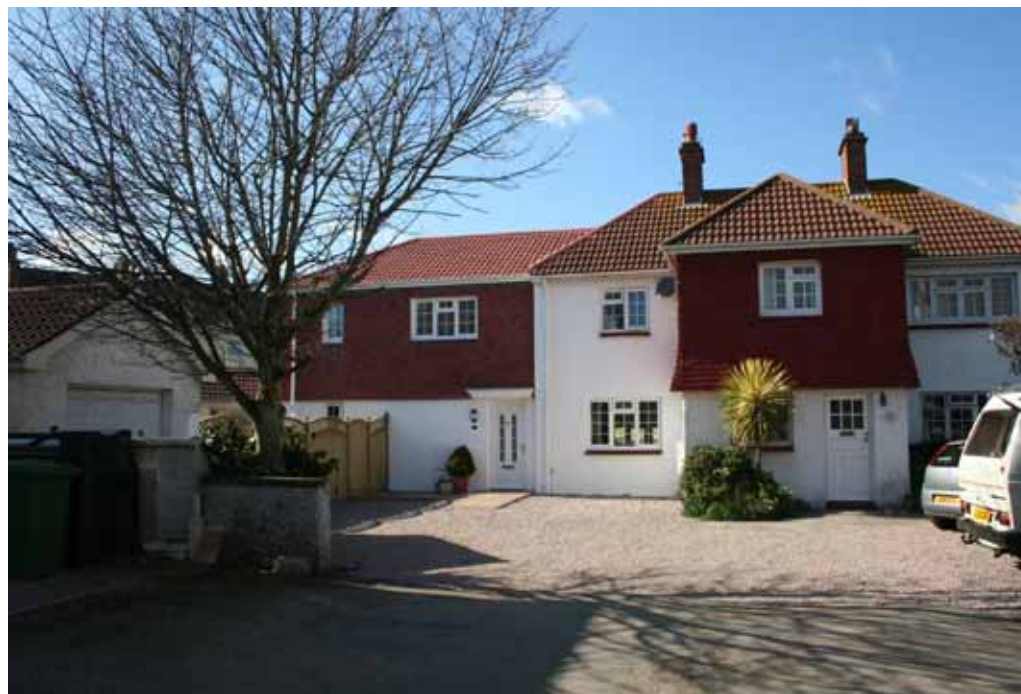
Images Right: Houses after completion.
